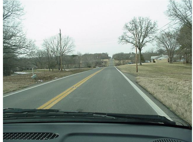
Photo No. 4 - Continuing northbound on KY 121.
