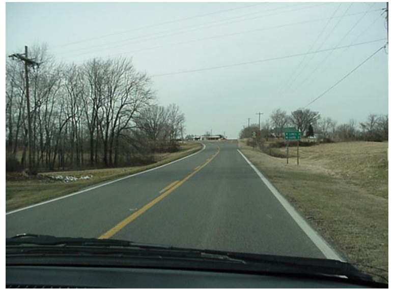
Photo No. 8 - KY 121 northbound, approaching intersection KY 440.
