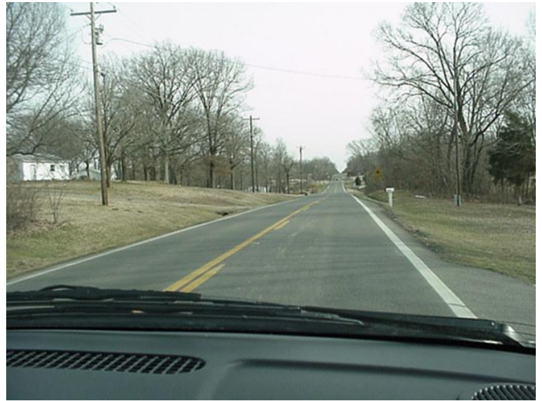
Photo No. 18 - KY 121 southbound through residential area.
