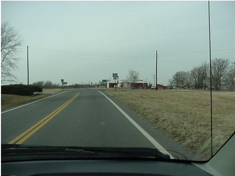
Photo No. 9 - KY 121 northbound, immediately north of intersection KY 440.
