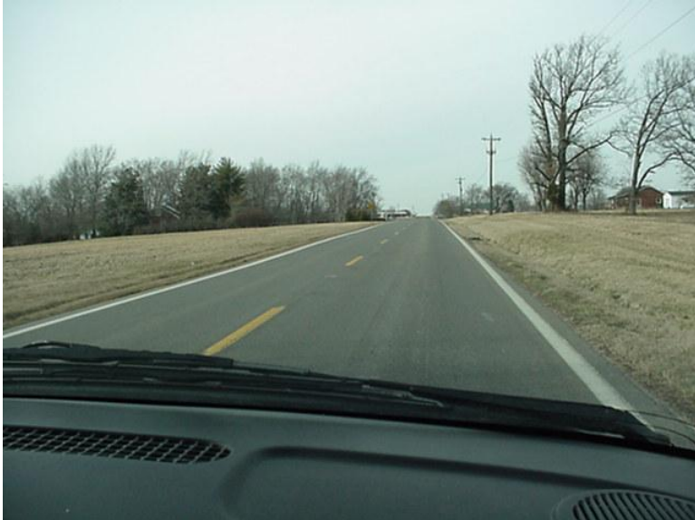
Photo No. 7 - KY 121 northbound, north of Jct. KY 1276.
