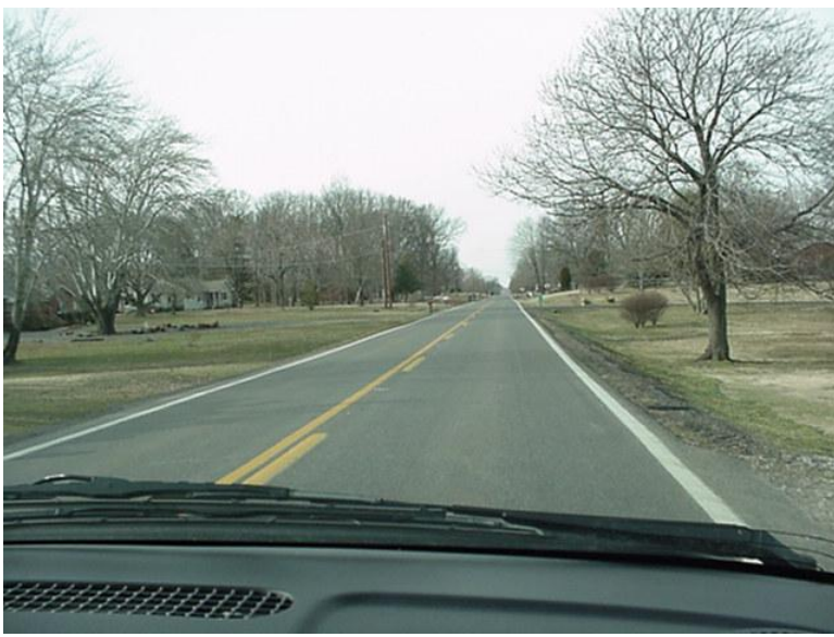
Photo No. 5 - KY 121 northbound travelling through residential area.
